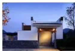
Household Energy Storage
