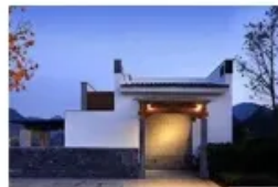
Household Energy Storage
